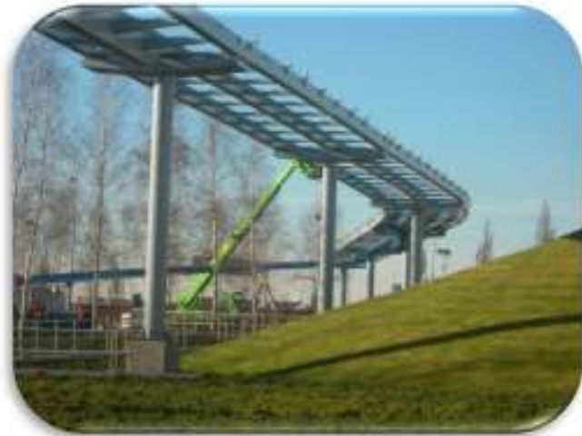
Heathrow Airport guideway construction
