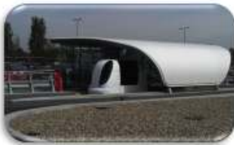
ULTra At-Grade Station
